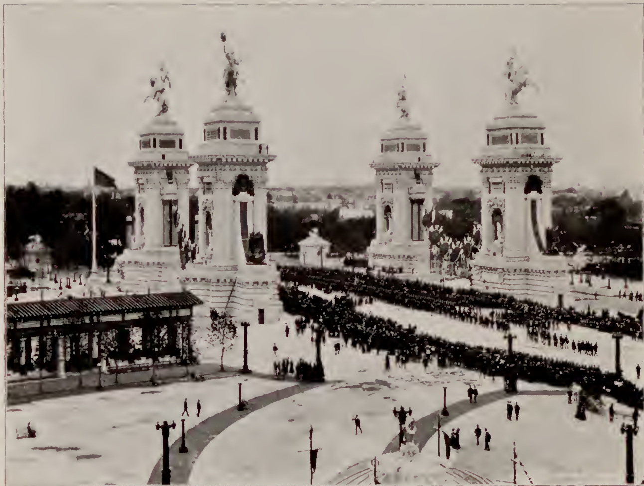
TRIUMPHAL BRIDGE ON DEDICATION DAY.—This view was taken as the Dedication Day procession reached the Esplanade. As the guests of honor, followed by U. S. Troops and National Guard regiments, passed over the Bridge, the sight was an impressive one.
